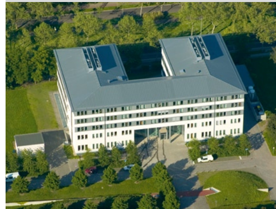
UFZ offices in Halle, Theodor-Lieser-Straße 4
